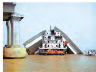
A Destroyed Bridge after a Ship Collision Accident
